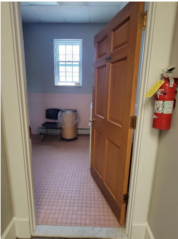
Entrance to Toilet Room
