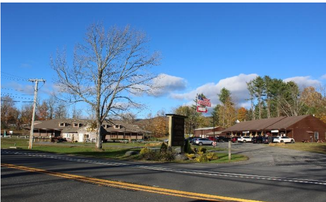
Commercial buildings extend along Route 7 until just north of Bailey Road.
