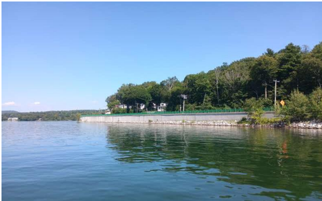
The sidewalk extends from Pontoosuc Lake Park into the town of Lanesborough, providing a bikeable and walkable route to the lake.
