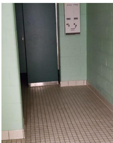
Entrance into the Toilet Room
