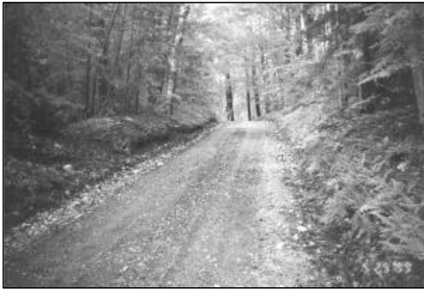
1. Before the project, Tyringham Road was narrow with steep banks and no formal ditches.
