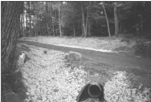
3. To improve the drainage, ditches were constructed on both sides of the road and culverts were used to direct water to stable outlets.
