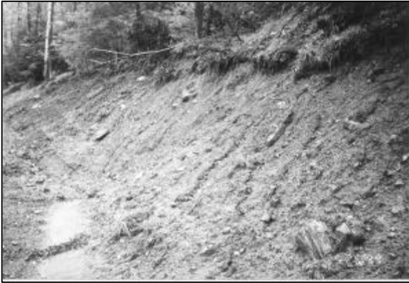
1. Before the project, the roadside bank was severely eroding which led to continual maintenance.
