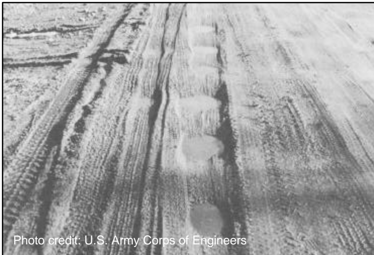
Corrugations on an unpaved roadway
