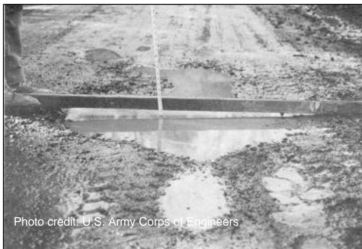
Pothole on an unpaved roadway
