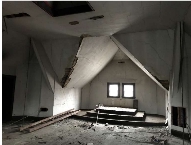
Deteriorating conditions of the attic space at the Deerfield Regional Senior Center (Franklin County). (Photo courtesy of the Town of Deerfield)
