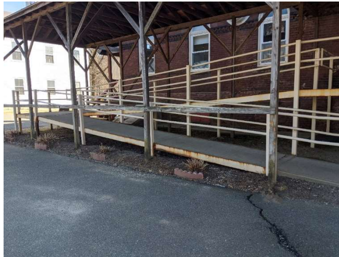
Rusting condition of the ramp at the Deerfield Regional Senior Center (Franklin County). (Photo courtesy of the Town of Deerfield)
