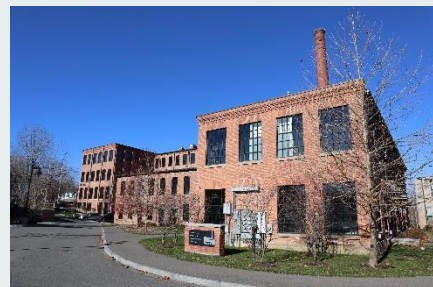
Cable Mills, Williamstown
