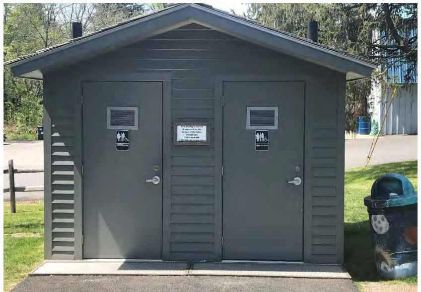
Example of public restroom facility along rail trail in Millerton, NY
