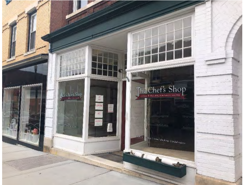
Improvements to vacant storefront façades can help attract new tenants
