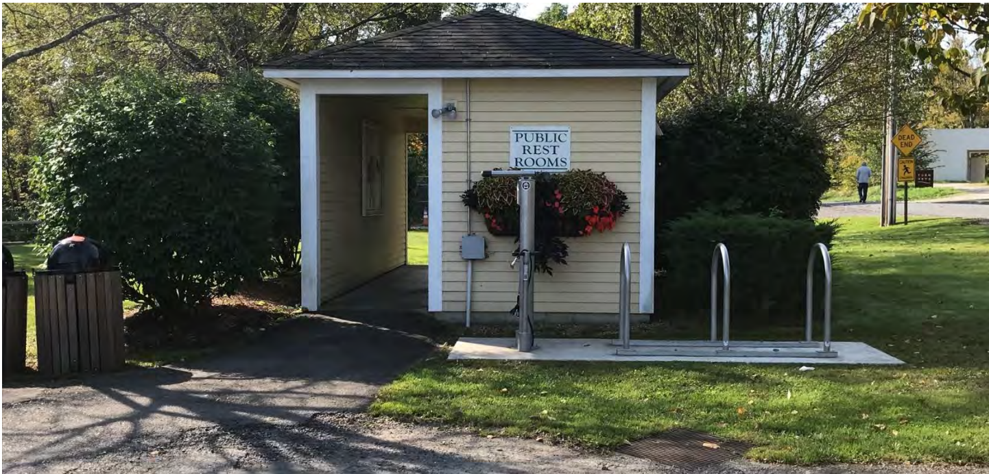
Example of public restroom construction and configuration in West Stockbridge, MA
