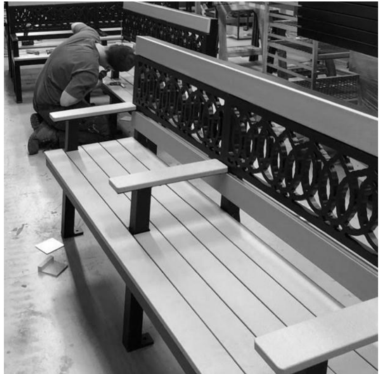
Themed benches being fabricated.
