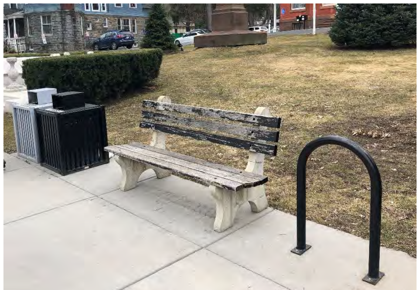
A dilapidated bench sits in front of the Town Hall campus
