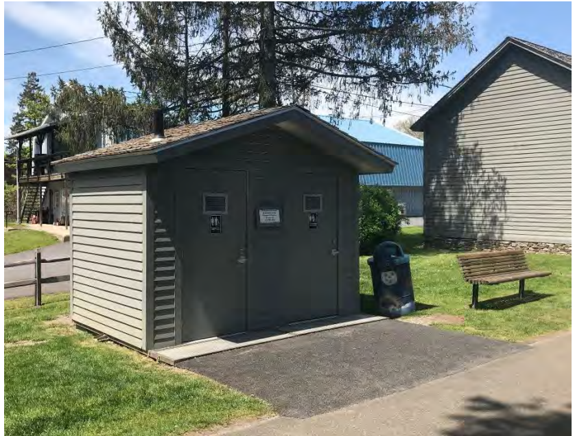
Example of public restroom facility along rail trail in Millerton, NY
