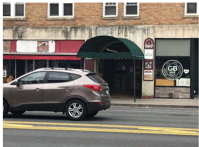
Damaged and unsightly awning on Main Street
