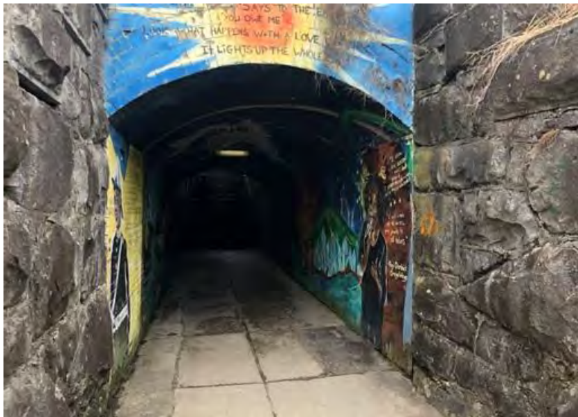
Pedestrian underpass leading from Town Hall to Castle Street and Castle Hill Avenue
