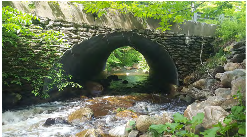
Figure 1c-1: Culvert carrying a stream under a road in Cheshire
