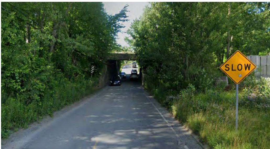
Figure 2c-1: Hubbard Avenue Rail overpass, seen approaching from the south.
