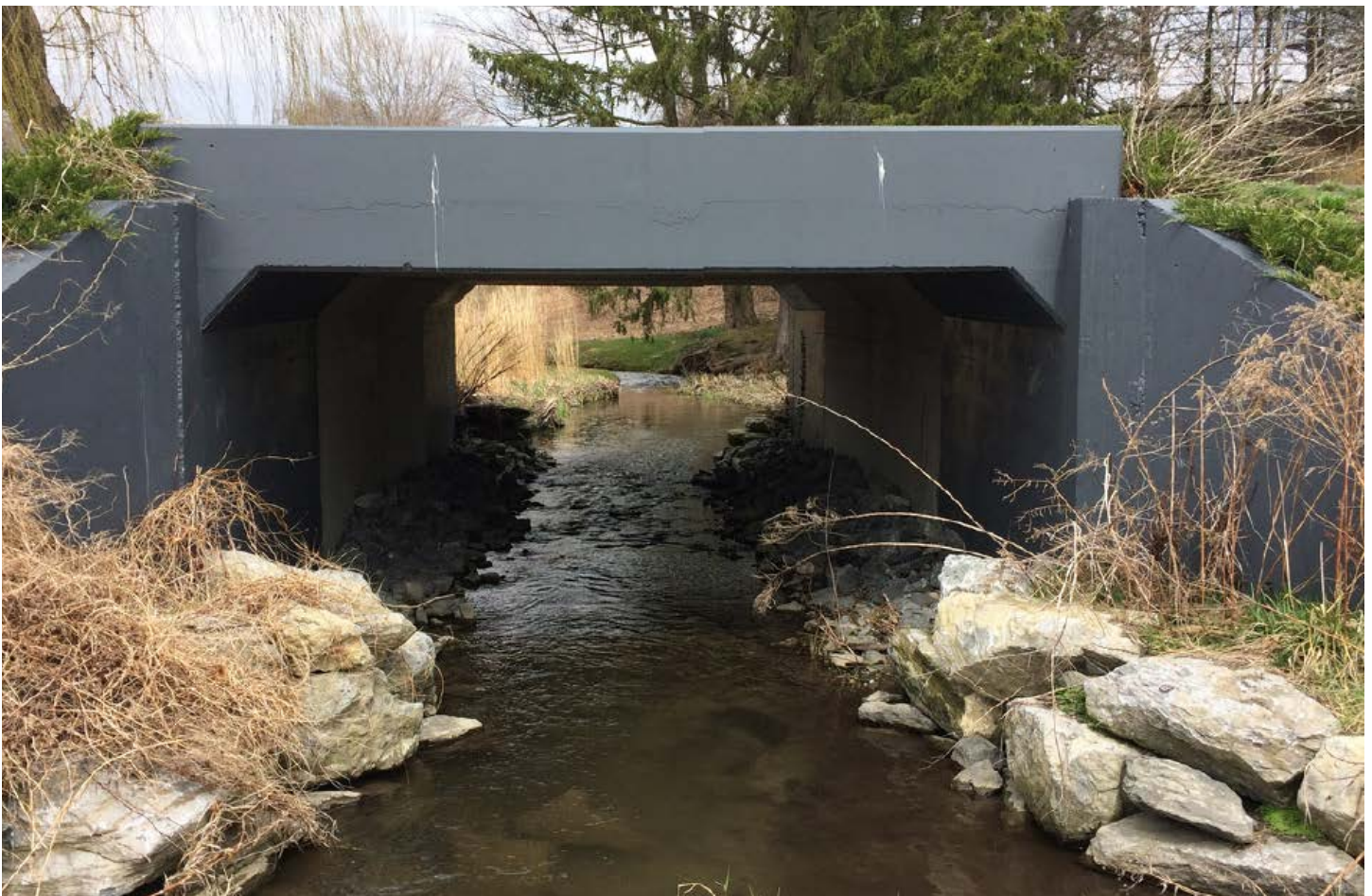
Figure 6c-2: A modern culvert built with adequate wildlife and stream crossing dimensions
