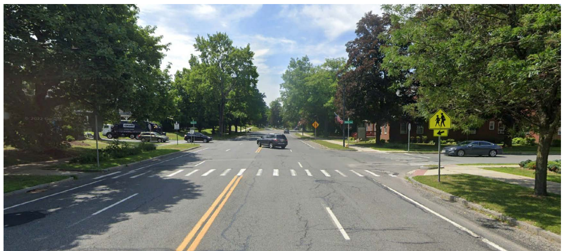
Figure 6b-1: Multiple-threat uncontrolled crossing on South Street in Pittsfield
