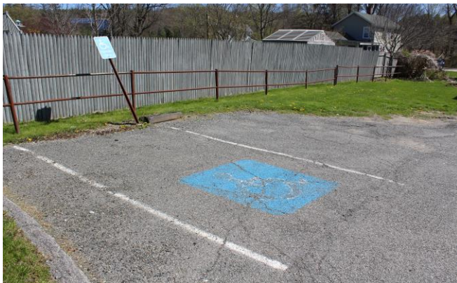
The paint and signage for the accessible parking is faded. There is also sufficient space to turn the spot to be van accessible.
