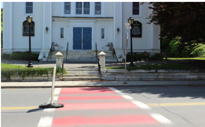
There are some crosswalks on Main Street that do not have curb ramps.
