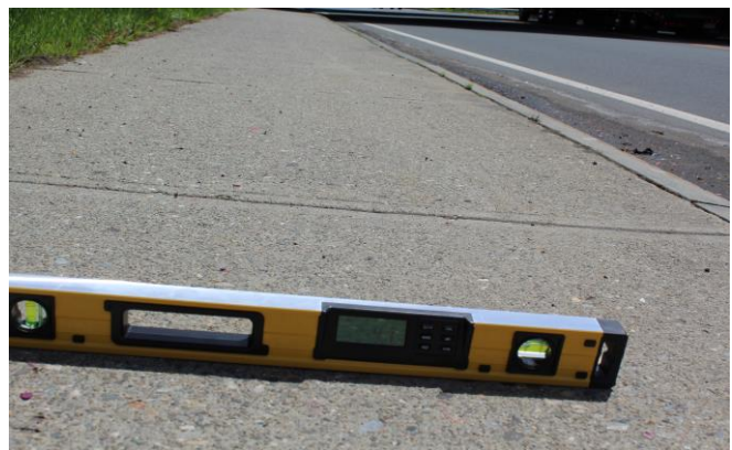
There are several locations on Housatonic Street and High Street where the cross slope exceeds the maximum 2% slope.
