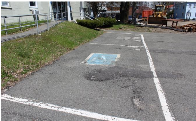
The accessible parking space's lines are fading and there is not signage.
