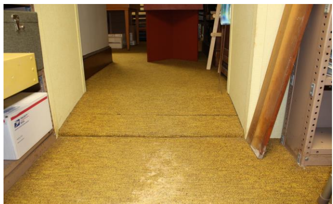
The change in level makes it difficult for someone to maneuver from one room to another in the basement.
