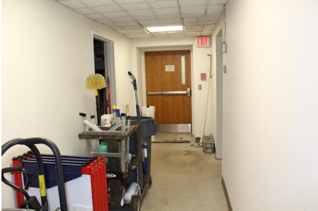
The hallways are cramped and do not allow someone in a wheelchair to turnaround. The floor features multiple broken tiles.
