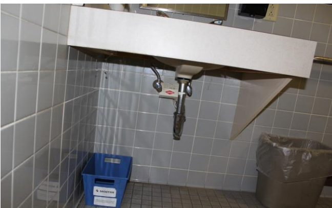
The bathrooms are compliant except for exposed pipes in the men's room.
