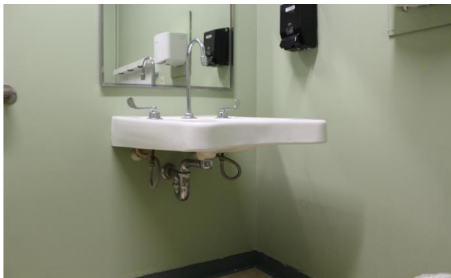
There are exposed pipes that should be covered.
