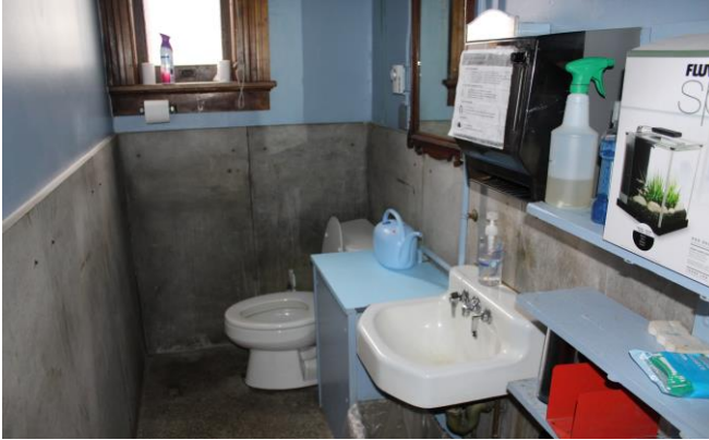
The staff bathroom is too narrow to comply with ADA standards.
