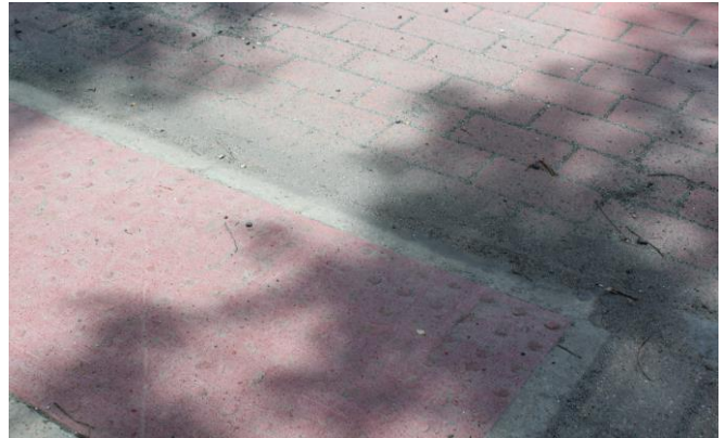
Many of the detectible footings have worn, most notably along Housatonic Street.
