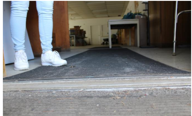
The transition into the building from the Railroad Street side is no longer smooth because the outside surface eroded.
