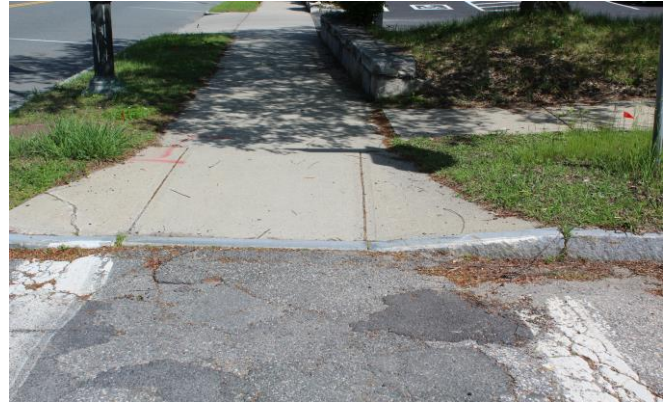
There are no curb ramps at some of the intersections with side roads in the downtown. The roads that the town has not reconstructed recently also have worn pavement, limiting accessibility.
