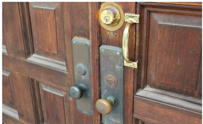
The town previously added a compliant handle to the front door to increase accessibility.
