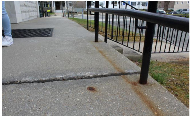
While still in compliance, a small lip is forming on the ADA ramp which the town should monitor.
