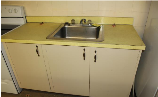
The sink is not equipped with the appropriate operable parts.
