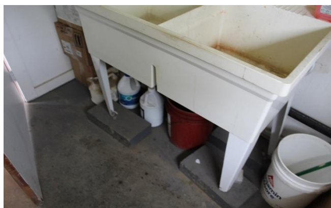
The sink does not provide proper knee clearance.
