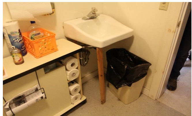
The sink does not provide sufficient knee clearances.
