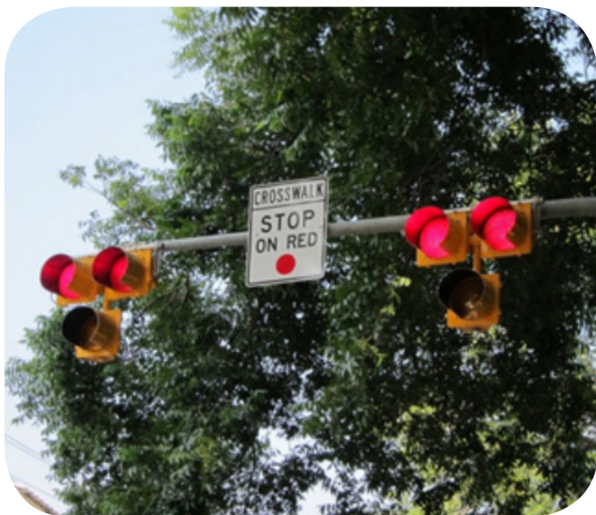
Pedestrian Hybrid Beacons have been found to reduce vehicle pedestrian crashes by 55% (Source: FHWA).
