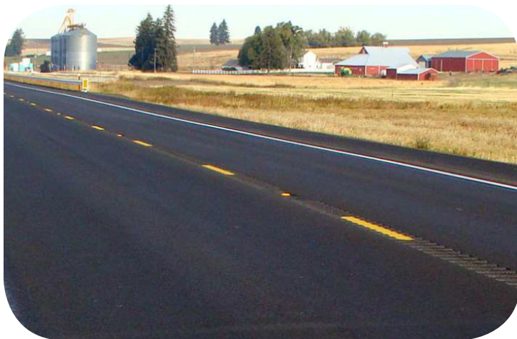
Centerline rumble strips (Source: FHWA).
