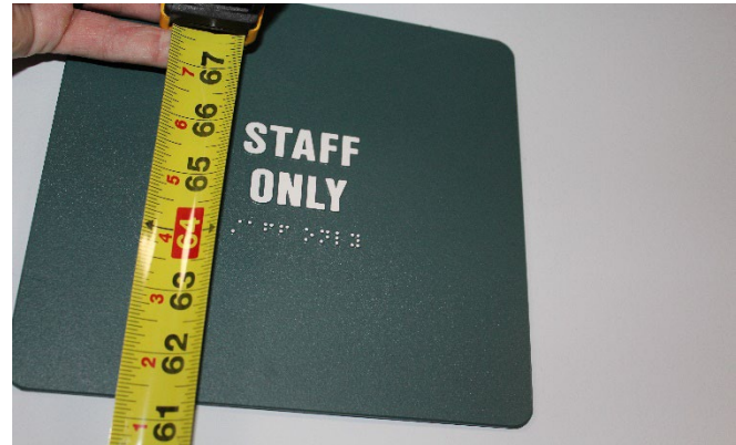
There is some inconsistency with signage throughout the building. MAAB requires signs to be 60" from the centerline of the sign to the ground.
