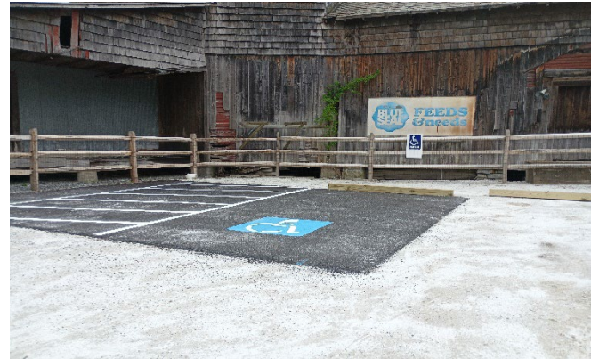
There is a paved accessible parking space at the park but the sign is not located at least 60" from the ground.
