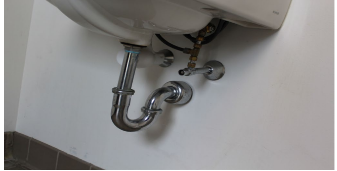
The pipes underneath the sink must be covered.
