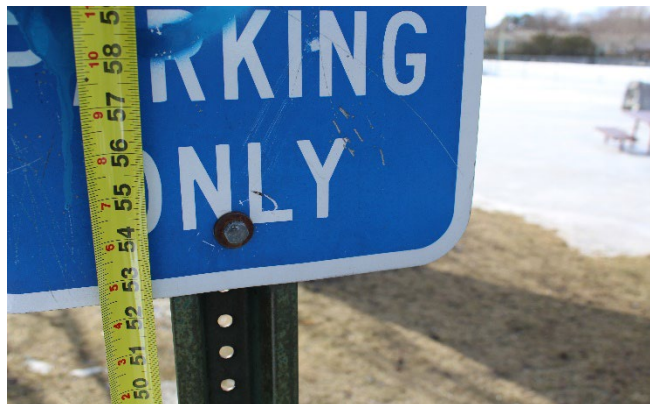
The signs must be at least 60" off the ground.
