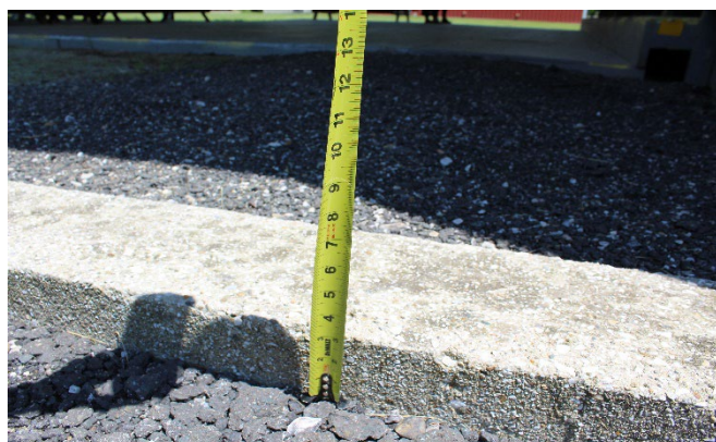
The gazebo is bordered by a stone that creates a significant change in level, rendering the gazebo inaccessible.
