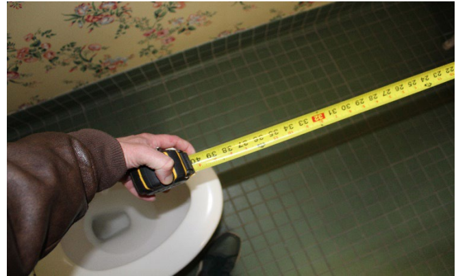
The radiator in the women's room limits the clear floor space in front of the toilet.
