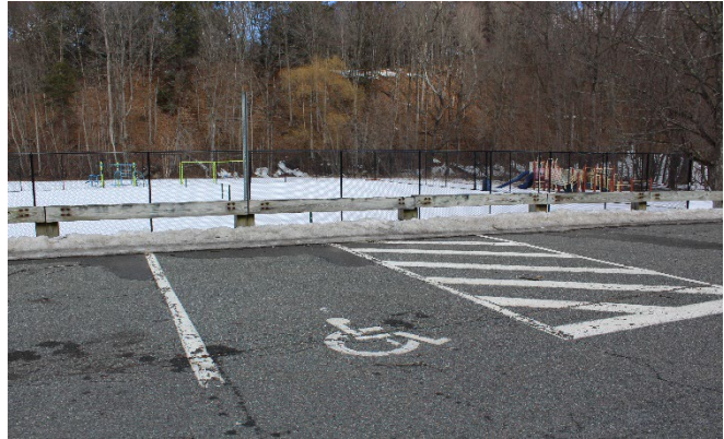
The northern accessible parking space is missing a sign and is not located closest to the accessible route to the playground.
