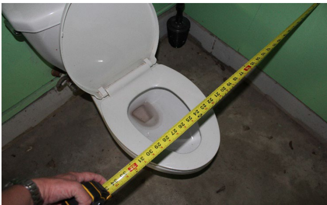
The toilets are located too far off the nearest wall and too close to the nearest fixture on the far side.
