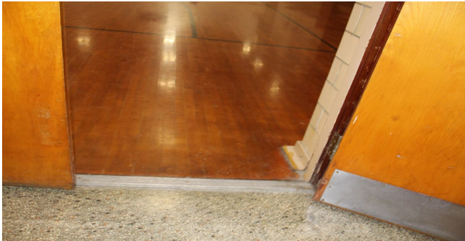
Thresholds throughout the building are not compliant.
