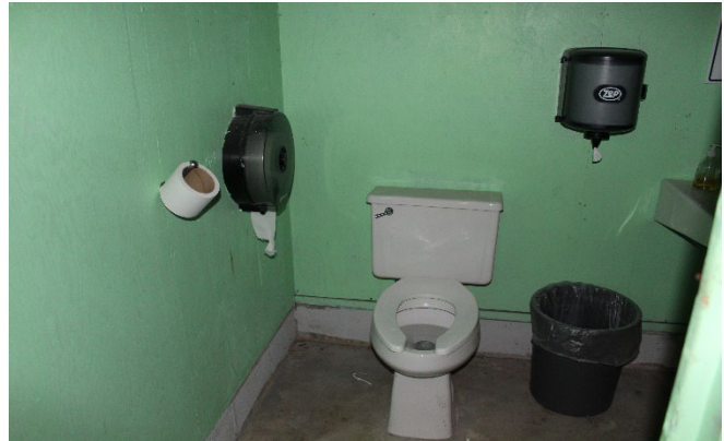
The toilet paper dispensers and the flush controls in the women's room are inappropriately located.
