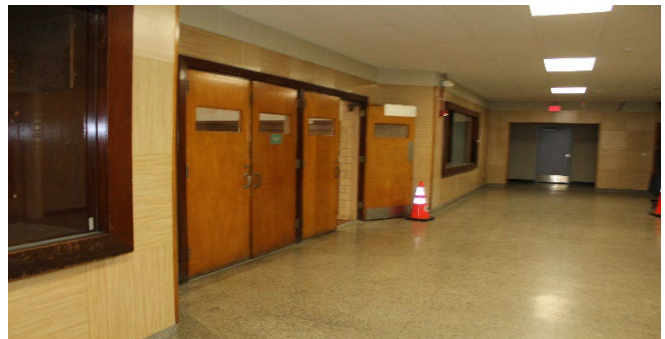
The doors to the gym provide sufficient space but have a threshold that needs to be lowered.
