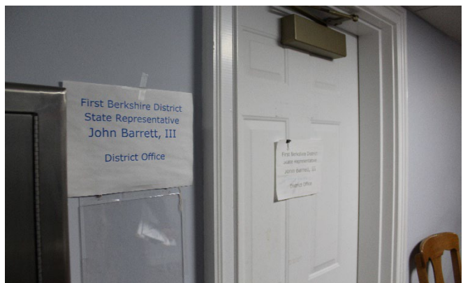
The sign to the state representative's office should be purchase and installed to comply with accessibility standards.
