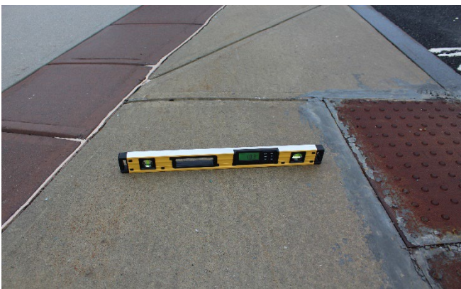
The slope of the curb ramp measures at 10.3%, which exceeds the 8.3% maximum.
