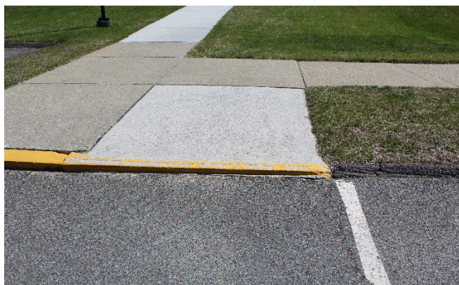
The curb cut is not compliant, limiting access from the accessible parking to the walkway into the building.
