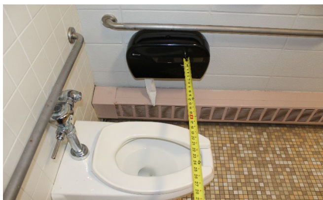
The centerline location of the toilet paper dispenser needs to be 7"-9" from the edge of the toilet seat.
