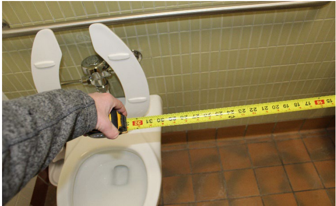
There is insufficient space from the far wall to the toilet.
