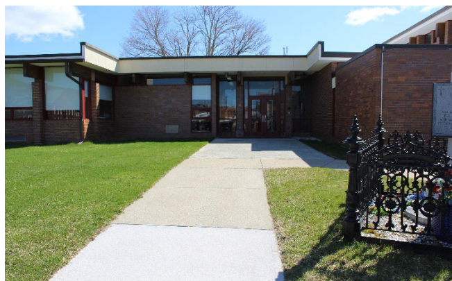
There is a walkway into the building but it does not have a compliant slope.
