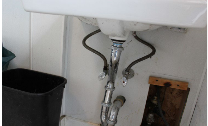
Bathroom piping should be insulated or guarded.
