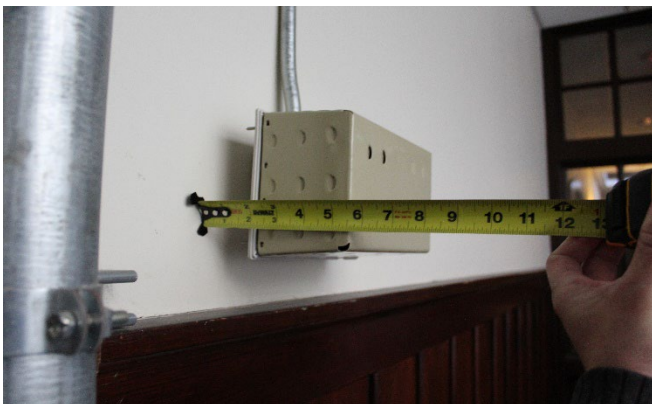
The control systems are protruding objects.
