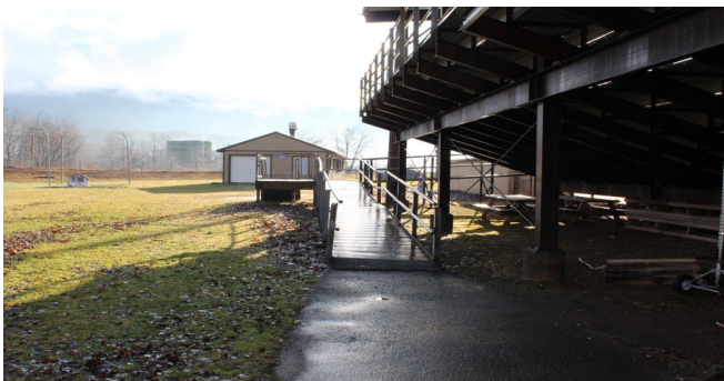
An accessible ramp provides access to the spectator seating.
