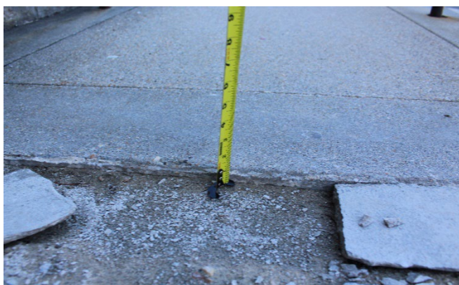
The concrete at the ramp is breaking down.
