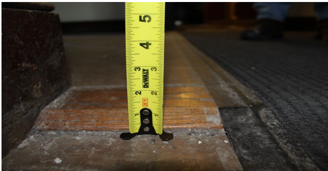
There are several thresholds that are not in compliance.
