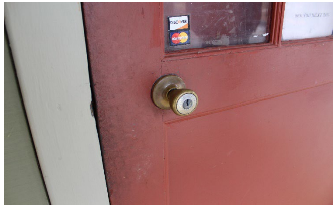
Door knobs are not in compliance with the 2010 ADA Standards.
