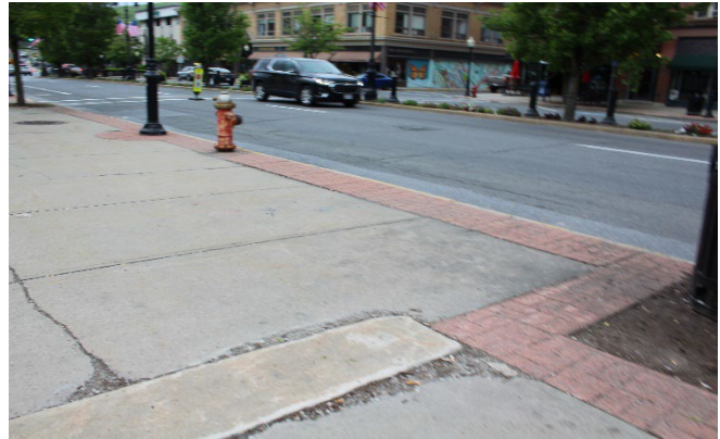
Sidewalks should be free of tripping hazards. Changes in level cannot exceed ¼".
