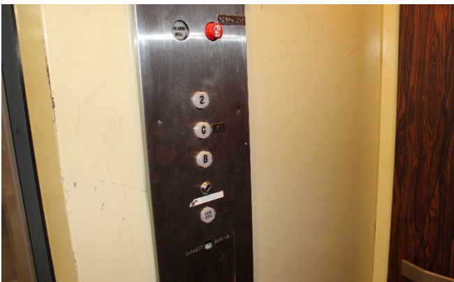
The elevator is missing braille and tactile control identifications as defined in Table 407.4.7.1.3 of the 2010 ADA Standards.
