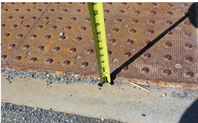
The tactile transition is exposed and there is not a smooth pathway to the front entrance.
