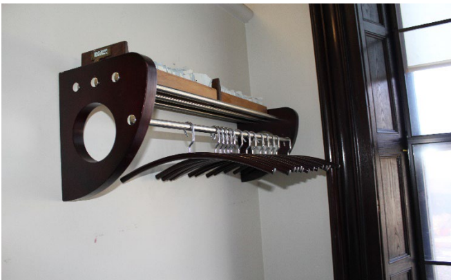
A coat rack is out of reach ranges.
