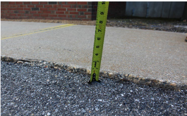
There is a change in level at the intersection between the parking lot and the curb ramp.
