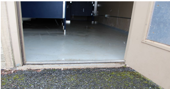
The thresholds to the bathroom exceed 1/4".
