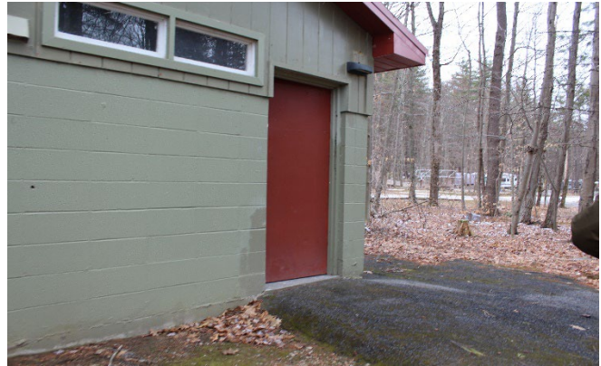
The pathway from the road to the accessible restroom does not have the appropriate grade.
