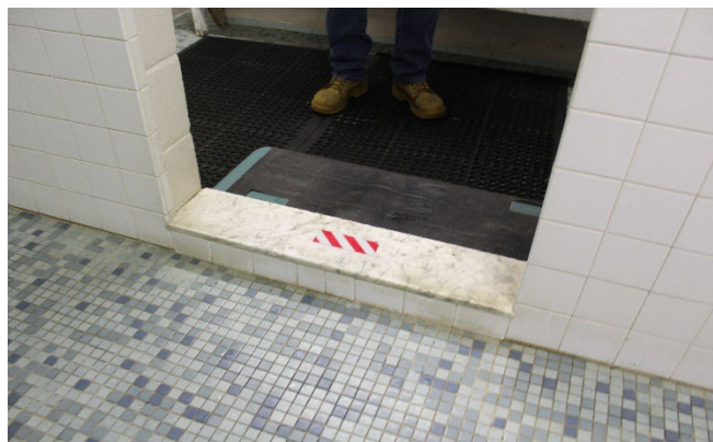
Steps throughout the locker room makes shower rooms and the sauna inaccessible.
