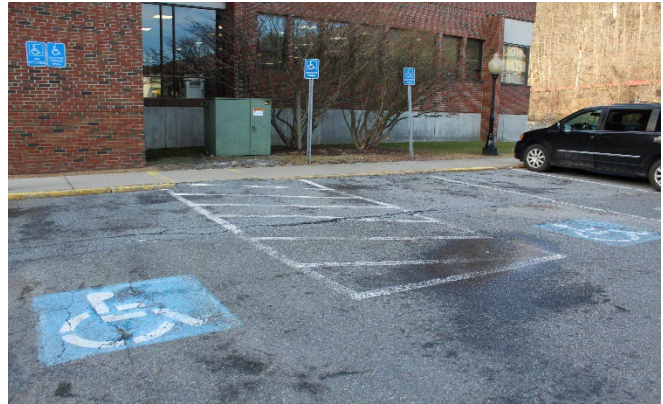
There is no aisle access in the accessible space to the far right.
