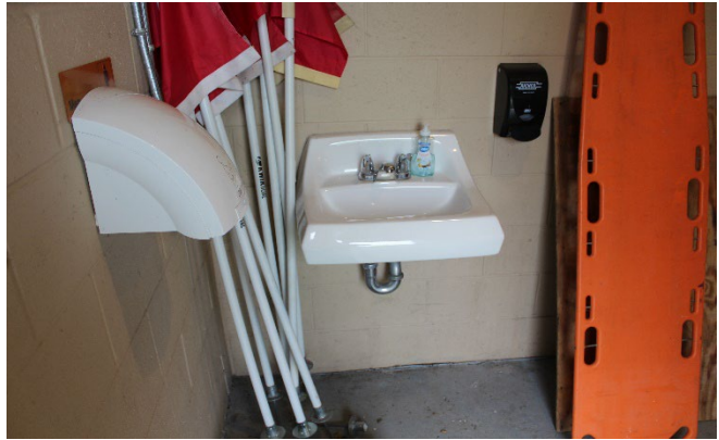
The hand dryer imposes on the path of travel to the sink.
