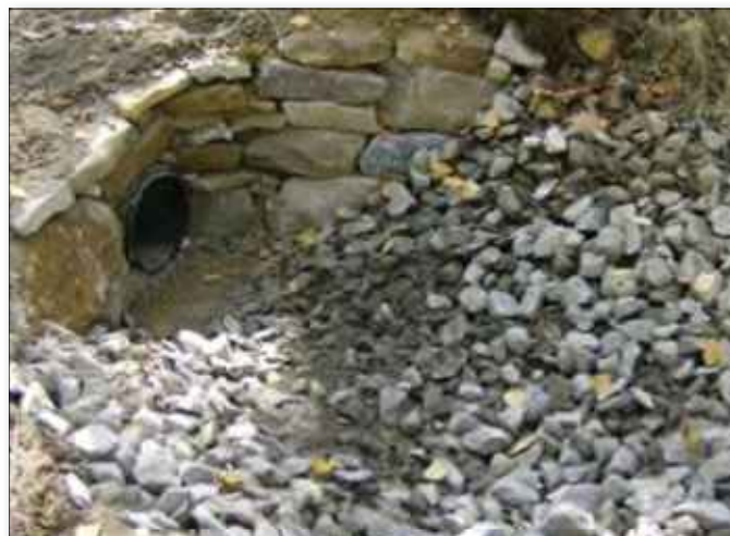
Stone-lined inlet to culvert.
