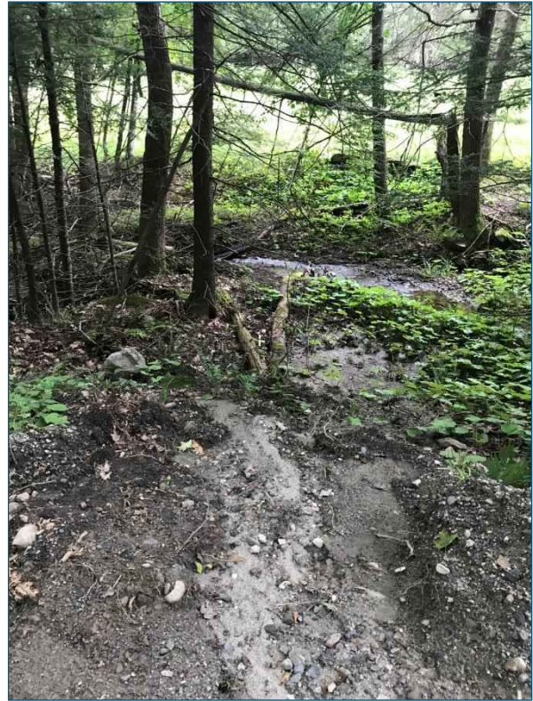
Without proper planning, stormwater will create a path off the road and into a stream.
