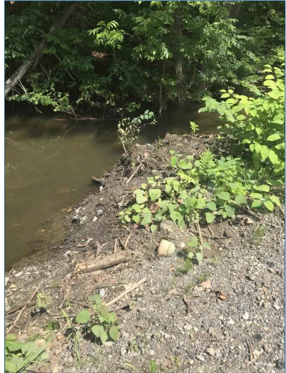
This wetland is so close to the road that it is difficult to manage stormwater and prevent road material from reaching it.
