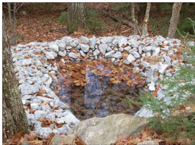
Plunge pool at outlet of culvert in woods.
