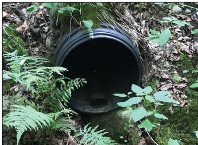
Round stormwater culvert outlet.
