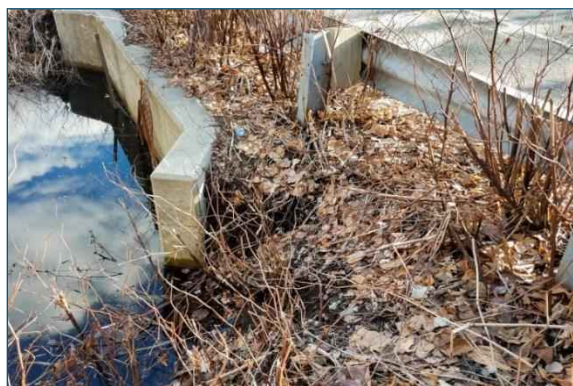
The knotweed surrounding this culvert is contributing to the loss of soil, which threatens both the roadway and the guardrail. Photo Credit: Brian Collieran Ecological Land Management
