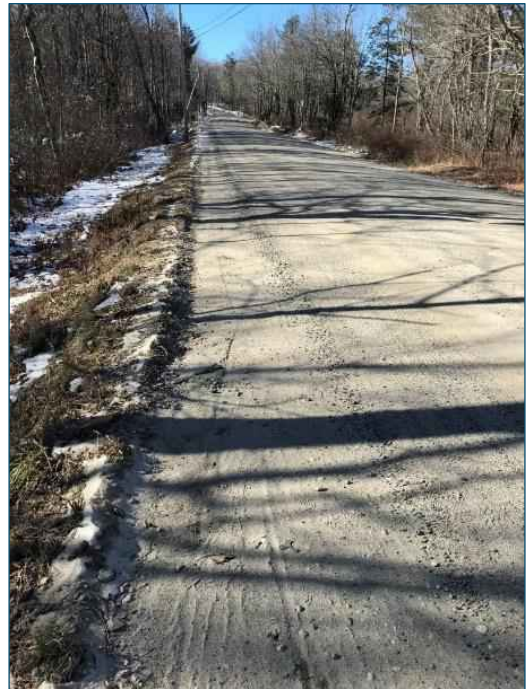
Road with grader berm.
