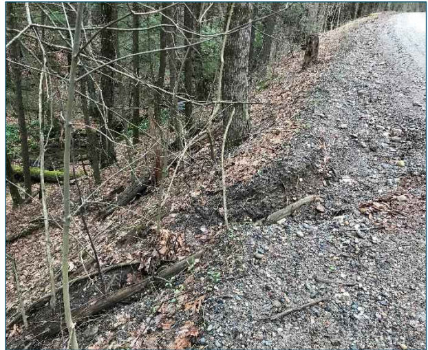
Gullies can form downhill as runoff finds its way off the road.
