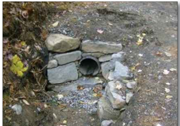
Stone headwall on a driveway culvert.
