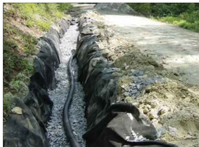
Underdrain under construction.
