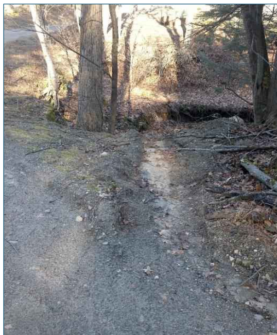
Turnout directed toward stream. Turnouts should be directed away from streams to allow water to infiltrate into the ground before reaching a stream.
