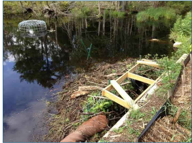
Fence and pipe system. Photo credit: Beaver Solutions.
