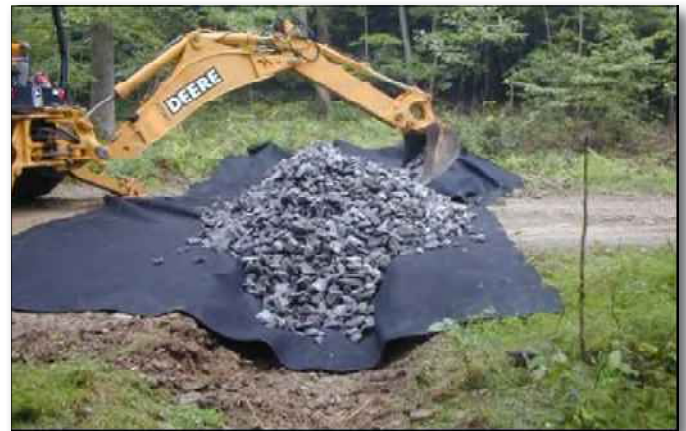
A small French mattress under construction.
