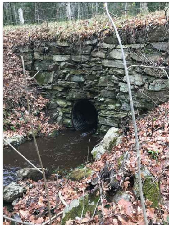
Fieldstone headwall on a stream-crossing culvert.
