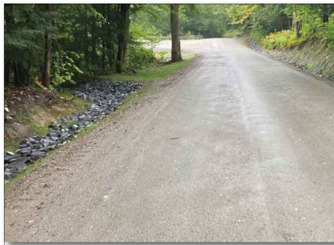
A stone-lined ditch (left side of road) ends in a stone-lined turnout.
