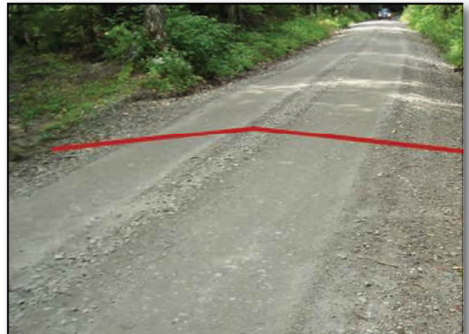
Road with centerline crown
