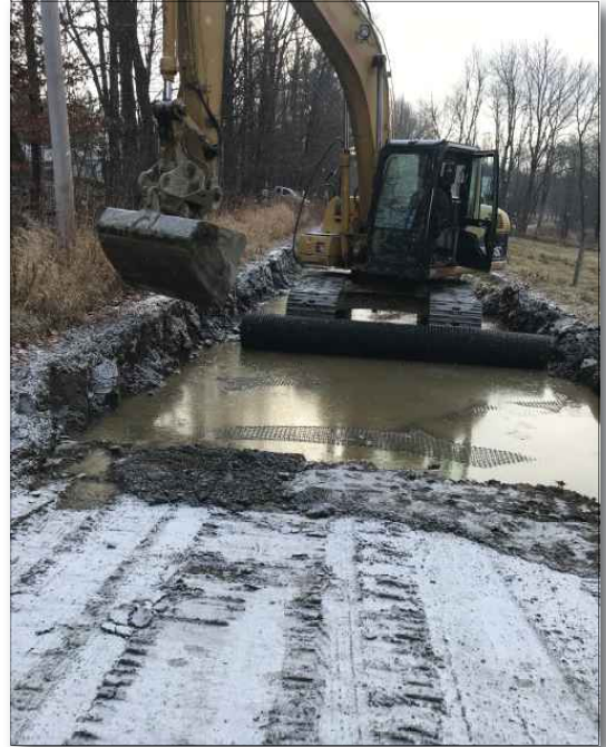
Geogrid being laid on a wet section of road in early winter.
