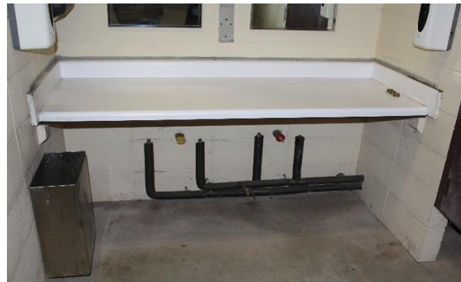
The pipes are appropriately covered, the trash can, and soap dispensers are at an appropriate height. However, the mirrors are slightly too high.
