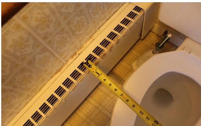
The heater infringes on the toilet.
