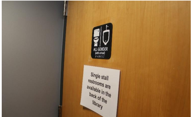
The sign on the accessible restroom are not located on the latch side and are outside of reach ranges.
