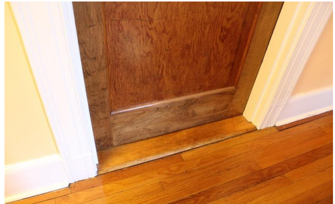
Thresholds throughout the building are not compliant.
