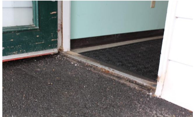
The thresholds at two of the entrances are deteriorating and create changes in levels above ¼."
