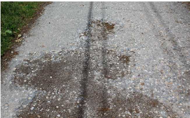
There are several areas along School Street where the concrete has deteriorated significantly and poses tripping hazards.
