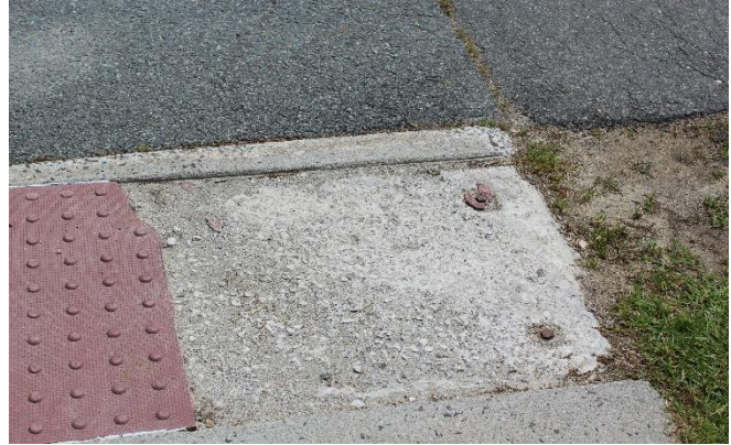
All of the tactile strips are damaged.
