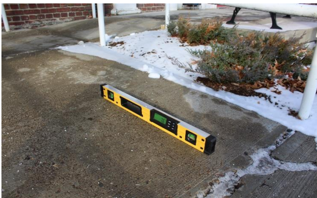
The front entrance measures at a slope of 9.1%, which is above standards.
