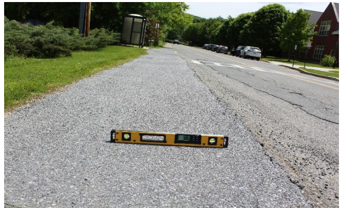
Excessive cross slopes are difficult to navigate.
