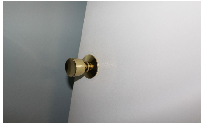
Door knobs are not accessible because they require
