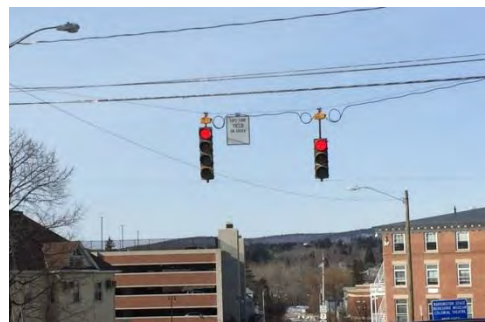
Image 6: Green ball is faded on R10-11 sign. Tyler Street west approach.
